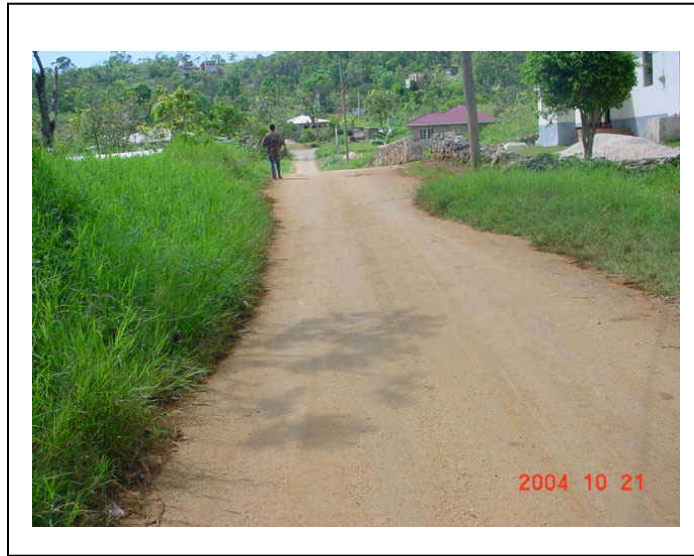
Plate 1 – Paved roadway constructed using Pave-Zyme basecourse
